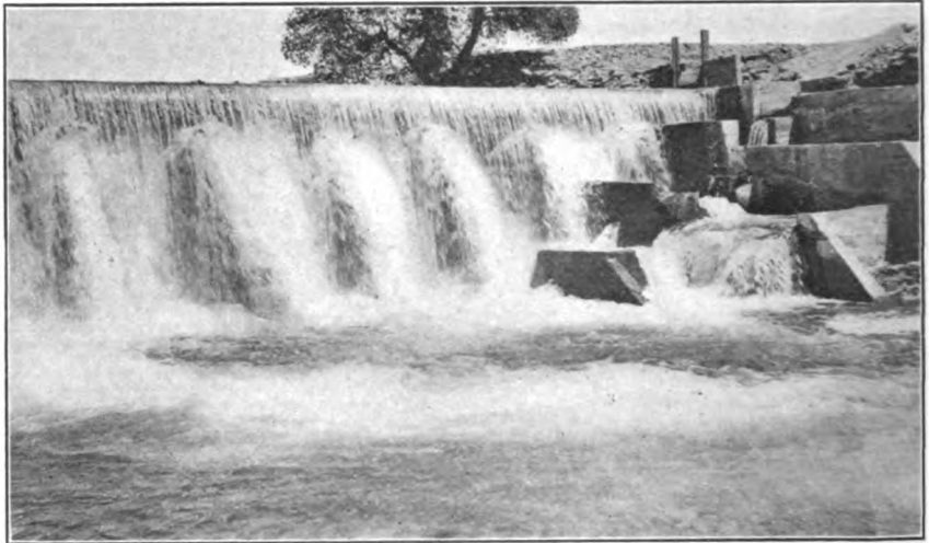
Fish-way over Clough Dam in Mill Creek, Tehama County.
