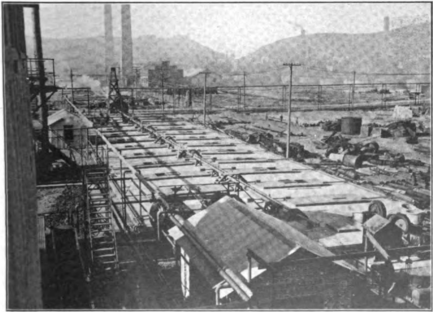
Fig. 75. Birdseye view of main separator of the Standard Oil Company plant at Richmond. The capacity is 20,000,000 gallons of waste per day. Photograph by A. M. Fairfield.
