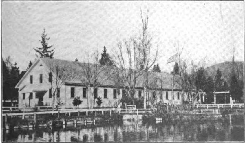
Fig. 43. Hatchery "A" at Sisson. Photograph by G. R. Field.
