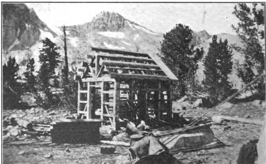
Fig. 50. New egg collecting station at Rae Lakes, showing the type of structure that must be erected to withstand the heavy snows at elevations above 10,000 feet. Photograph by F. H. Shebley.
