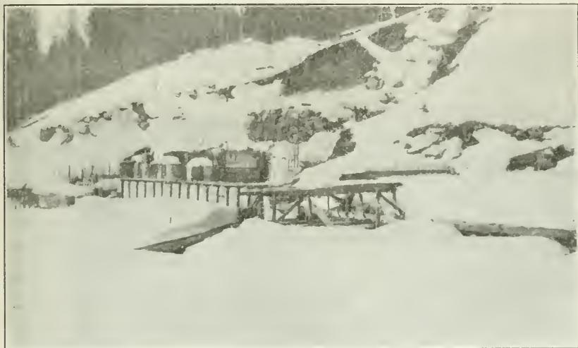
FIG. 10. Eyeing house and tank at Canyon Dam, Lake Almanor, Plumas County, April, 1919. Spawning operations must be begun under such conditions as these. Photograph by S. Campbell.
