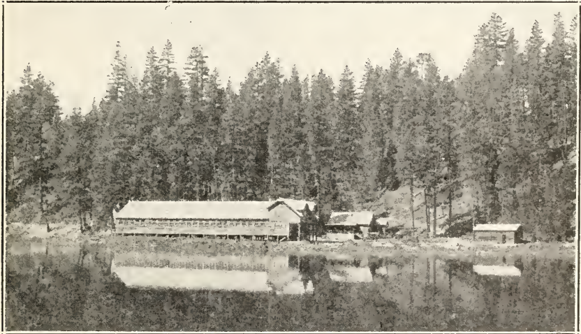
FIG. 15. The new Burney Creek Fish Hatchery.
