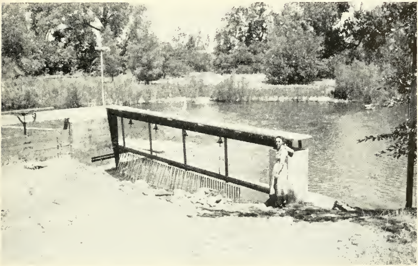
FIGURE 9. Mill Creek electric fish screen
