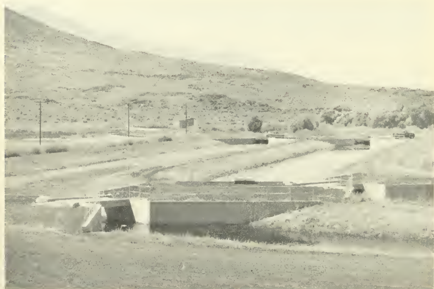
View showing a portion of the pond system at the new Fish Springs Hatchery located near Bigpine, Inyo County. Two parallel series of ponds are employed, each series a little over 1,700 feet long. The ponds have a total capacity of nearly 1,000,000 catchable trout annually. The Fish Springs Hatchery is ideally situated to serve an area of extremely heavy fishing pressure.
