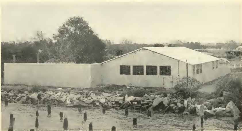
The new Delta Field Base, on the San Joaquin River near the Antioch Bridge, was built during 1951 with Wildlife Conservation Board funds. The building contains adequate storage and working space for the various delta activities of the department, including berths for three boats, the Striper , Rainbow , and Minnow .
