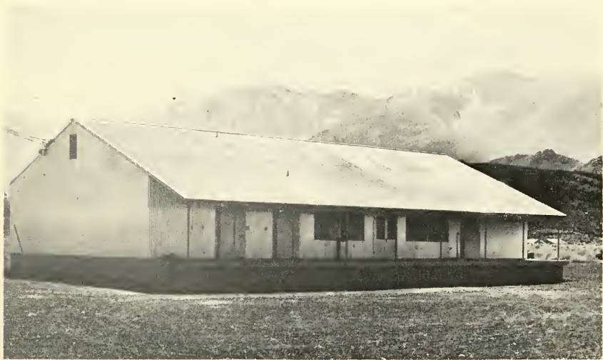
The food preparation building, Fish Springs Hatchery. With a refrigerated storage capacity of 100,000 pounds of frozen food and utilizing the latest ice-making and food-processing equipment, this building will go a long way in reducing the manpower requirements at this installation. A building of similar style houses an office for the foreman, the shop and repair department, vehicle storage and public rest rooms. The hatchery represents an investment of nearly $400,000 of Wildlife Conservation Board funds.
