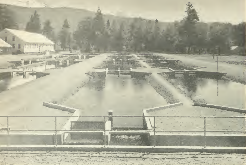
Rehabilitation of the Mt. Shasta Hatchery, in continuous operation since 1888 and California's oldest fish-rearing station, was completed early in 1952. Modernization of this old hatchery to fit it into a new hatchery expansion program was made possible through allocation of $240,000 from the Wildlife Conservation Board. Improvements include 16 new earth-fill raceway ponds with concrete dividing dams, the new 124-trough hatchery building (left) and a new food preparation building. This is a fine example of modernization of an old unit to fit a new program.
