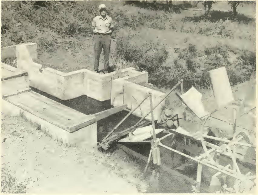
This is a perforated plate fish screen with gear drive. The perforated plate has been inserted into the downstream end of a form originally built for a revolving drum screen. Young trout and salmon descend the irrigation ditch as far as the screen, then are diverted back to the parent stream through the bypass channel directly in front of Fish Hatchery Foreman E. W. Murphey, the inventor of the perforated plate screen. Siskiyou County, 1951.
