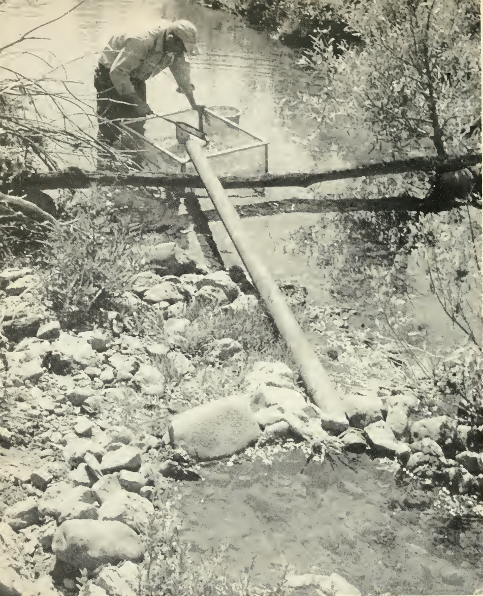
Fish rescue trap designed by G. R. Holman. The whole flow of a small tributary stream which has dried up in its lower portion is diverted into a mesh box placed at the terminal end of the flow. The downstream migrating fingerlings are trapped and removed each morning. Fish rescue is an incidental program of the crew working in the North Coast area. During May and June, 1952, a total of 19,400 steelhead and 3,998 silver salmon was rescued.
