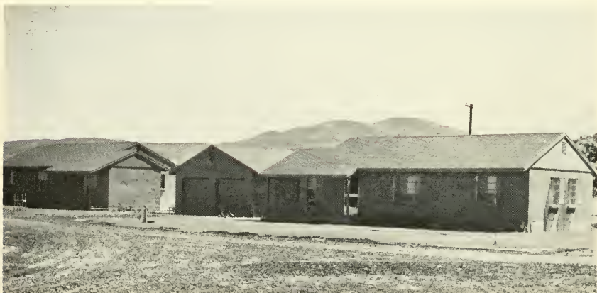
Two of the six pumice-block dwellings at the new Fish Springs Hatchery. It is necessary for the department to provide living quarters at remote stations.
