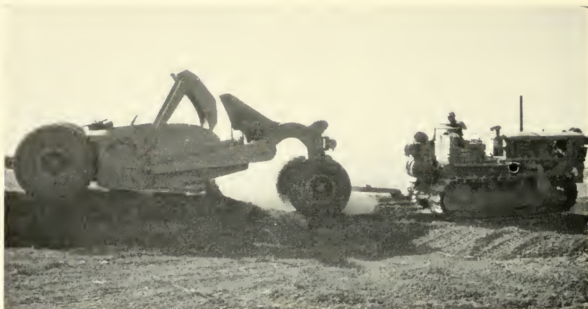
To provide ponds for waterfowl often requires construction of levees on management areas. Such work requires the use of heavy equipment.
