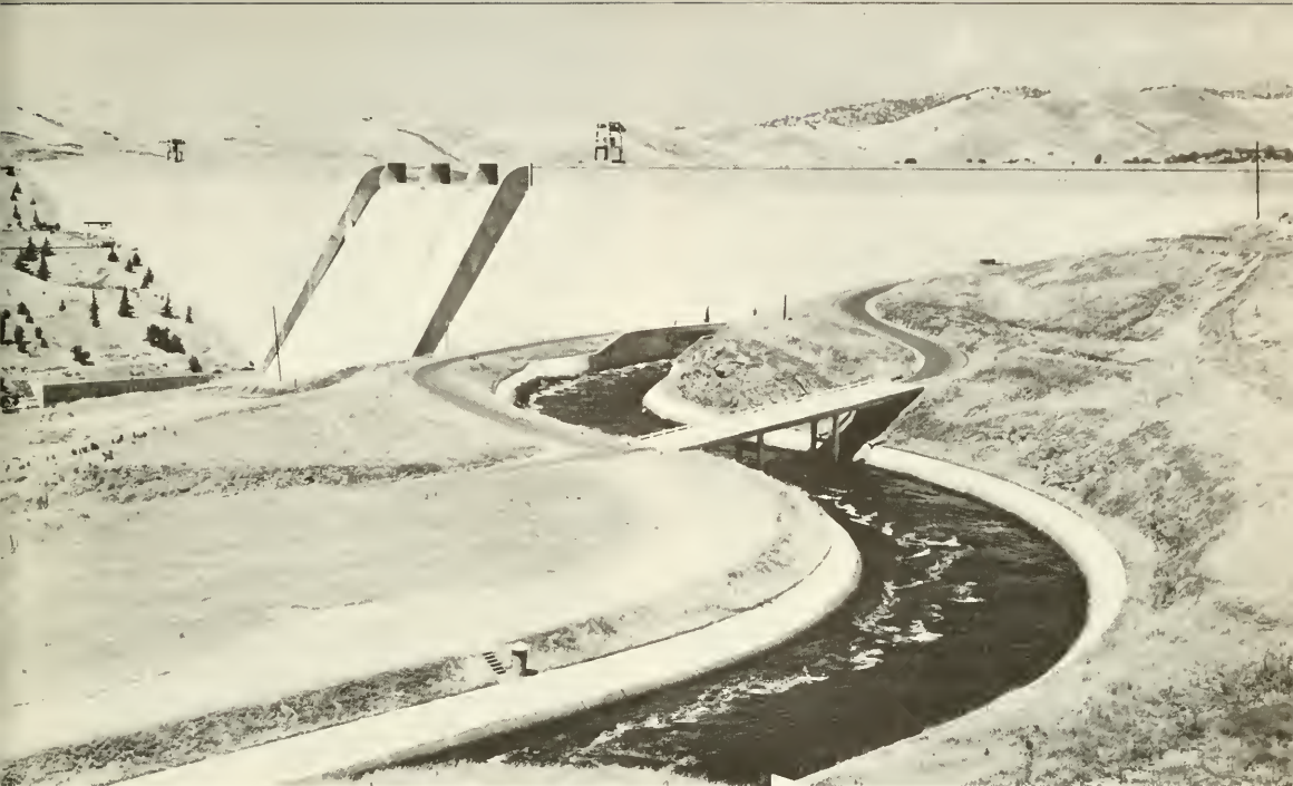
Water diverted from Friant Dam, background, has left salmon high and dry during spawning runs up the San Joaquin River. The department was seeking water for salmon at a State Water Rights Board hearing which began at the end of the biennium.
