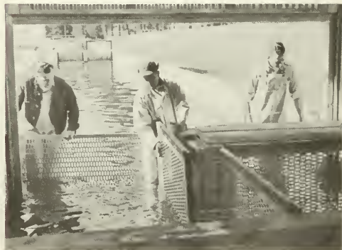
Perforated aluminum grates for pushing brood fish into the spawning house at Mt. Shasta Hatchery.
