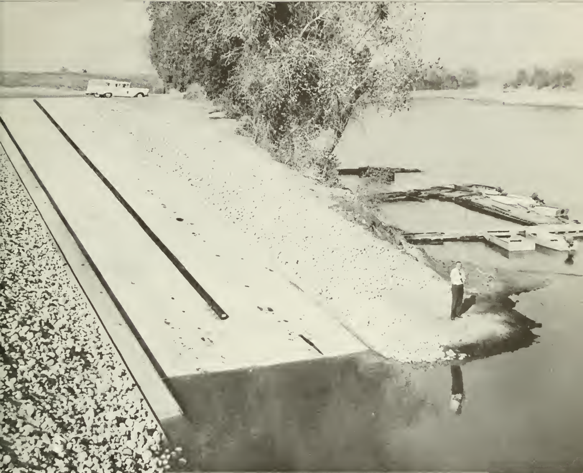
Typical of access sites provided by Wildlife Conservation Board funds is this one on the Feather River near Boyd's Pump. Under construction in the biennium, the ramp is 22 feet wide and has a two-foot walkway down the left side. Boat docks were built by local sportsmen.
