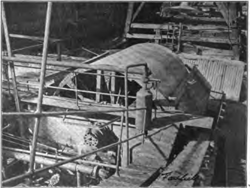
Fig. 78. Oliver filter at the Potrero plant of the Pacific Gas and Electric Company, San Francisco. Photograph by A. M. Fairfield.
