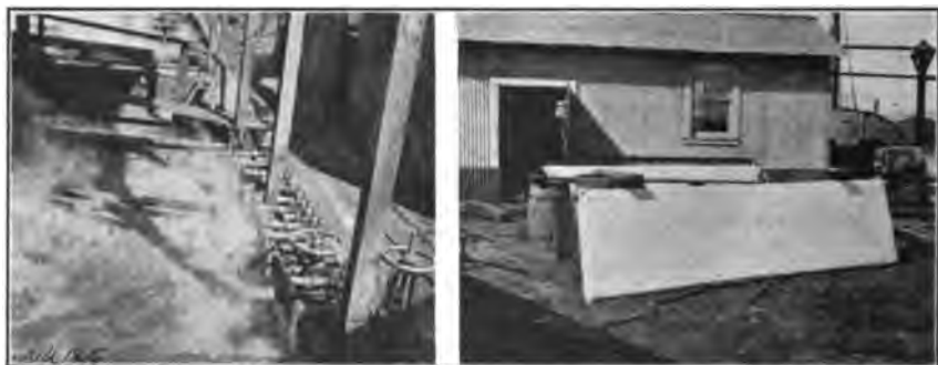
Fig. 81. Butters filter and filter leaf at plant of Pacific Gas and Electric Company at Oakland. Photograph by A. M. Fairfield.
