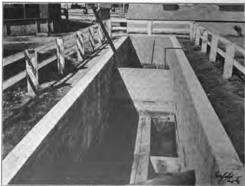
Fig. 84. Southern Pacific oil trap at San José, 10' x 50' x 18'. There are similar traps at San Luis Obispo, Watsonville Junction and San Francisco. Photograph by A. M. Fairfield.
