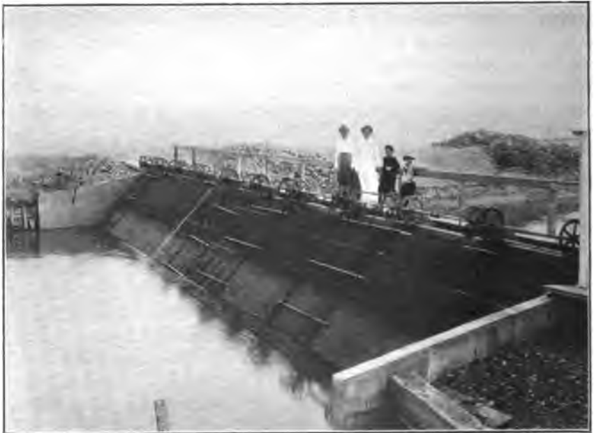
Screen of Sacramento Valley West Side Canal Co., in Stony Creek, Glenn County. Seventy feet long and sixteen feet deep.
