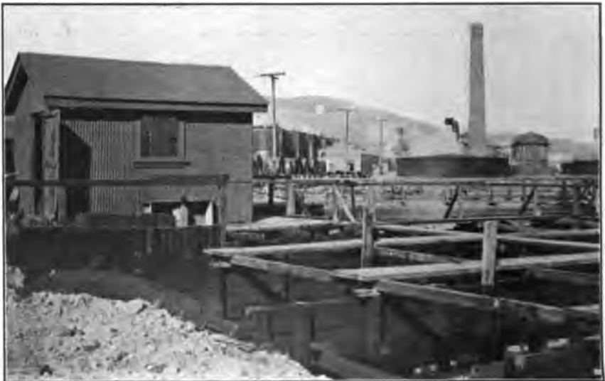
Fig. 76. Detail view of baffles of the Standard Oil Company plant at Richmond. The oil collects behind the baffles and is skimmed and pumped back into the separator. Photograph by A. M. Fairfield.
