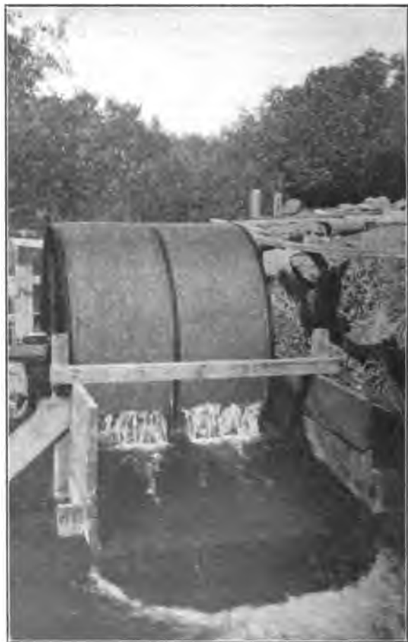
Fig. 33. Screen installed in an irrigating ditch near Edgewood, Siskiyou County. Fish are prevented from entering this ditch, but the flow of water is unhampered. Photograph by A. E. Culver.
