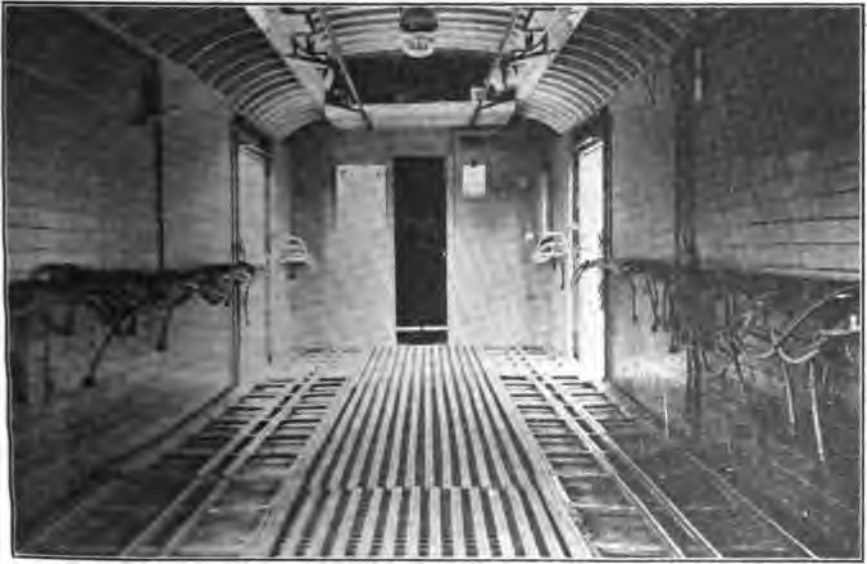
Fig. 21. Interior of fish car No. 2, showing aerating apparatus.
