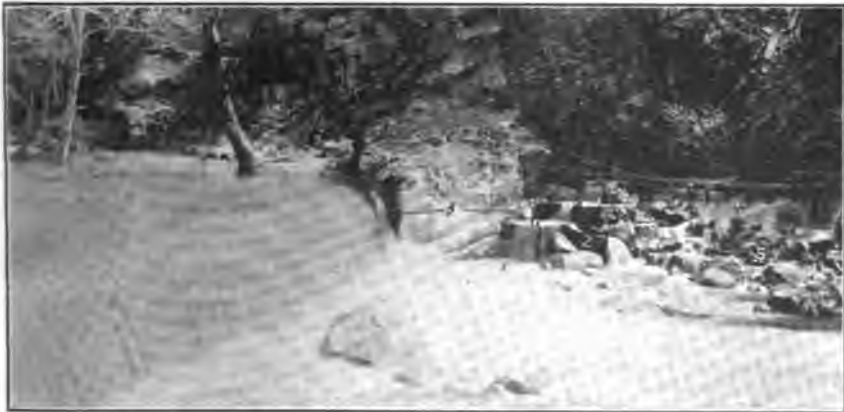
Fig. 40. Fishway at Bonally Dam, on the Salmon River, Siskiyou County. Photograph by I. Eldredge.
