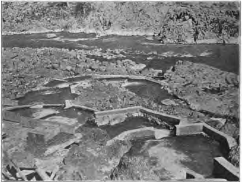
Fig. 41. Snow Mountain Dam Fishway, on south fork of Eel River, Mendocino County. Photograph by H. C. Bryant.
