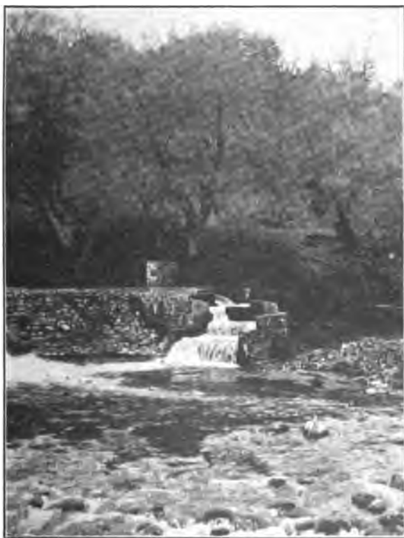
Fig. 39. Fish ladder constructed by Northern California Power Company on Butte Creek, Tehama County. Photograph by A. E. Culver.
