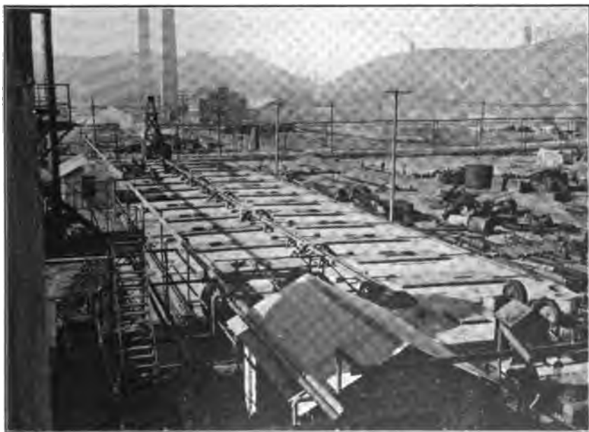
Fig. 75. Birdseye view of main separator of the Standard Oil Company plant at Richmond. The capacity is 20,000,000 gallons of waste per day. Photograph by A. M. Fairfield.
