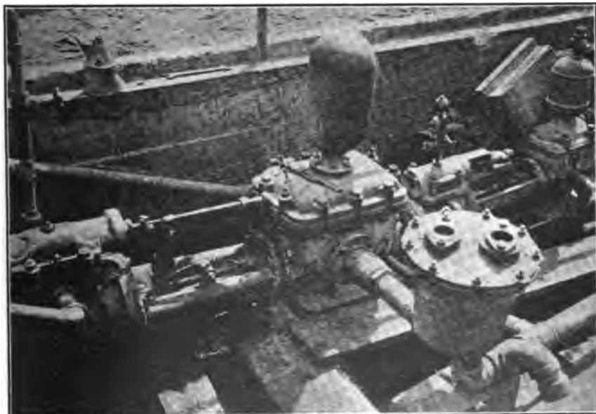
Fig. 82. Pump for waste oil recovery in oil trap of the Southern Pacific at West Oakland. Photograph by A. M. Fairfield.
