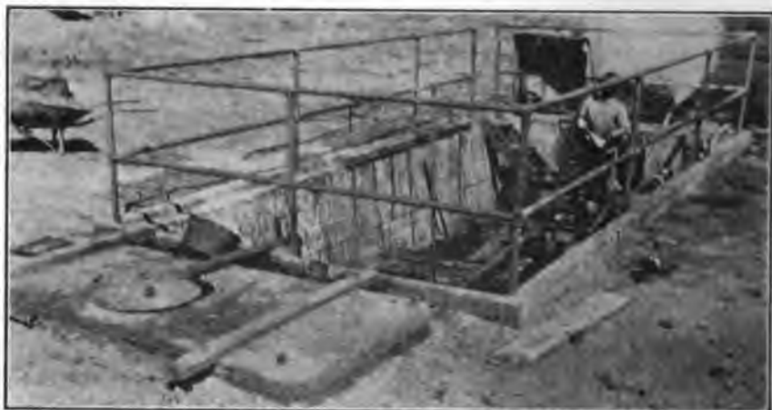
Fig. 83. Oil trap of the Southern Pacific at West Oakland. Photograph by A. M. Fairfield.
