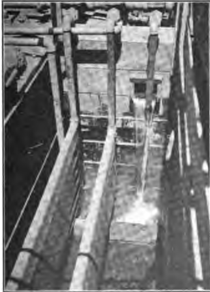
Fig. 80. Butters filter at Santa Rosa. Handles lampblack from 375,000 cubic feet of gas per day. Photograph by A. M. Fairfield.
