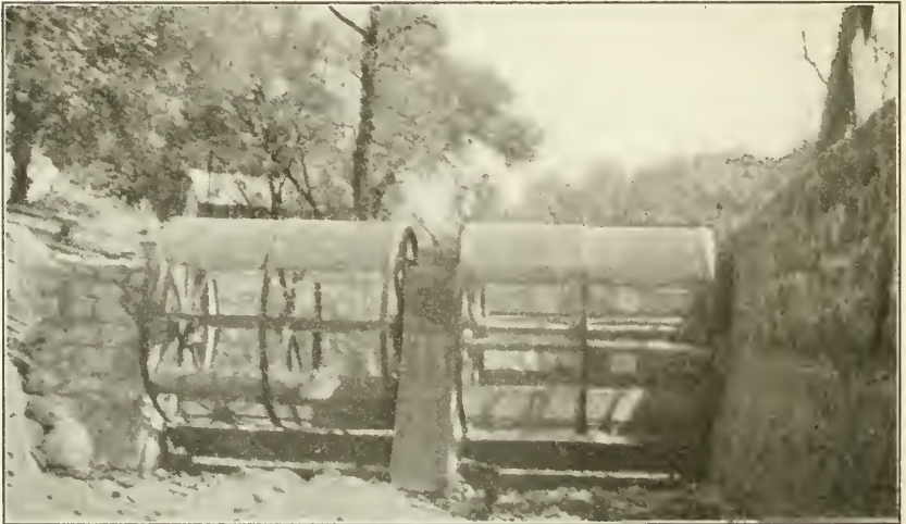
Fig. 42. Screen of Northern California Power Company at Inskips, Tehama County. Photograph by A. E. Culver.
