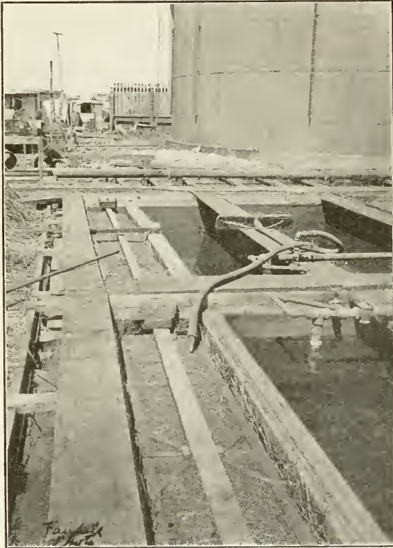
Fig. 77. Superior type of straw filter of the Pacific Gas and Electric Company at Vallejo. Photograph by A. M. Fairfield.
