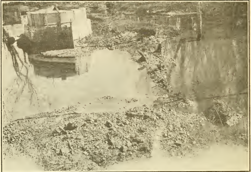
FIG. 30. Sump of Sacramento Gas Company on March 1, 1922. Flood waters have opened sump and lampblack is passing into Sacramento River. Photograph by A. M. Fairfield.
