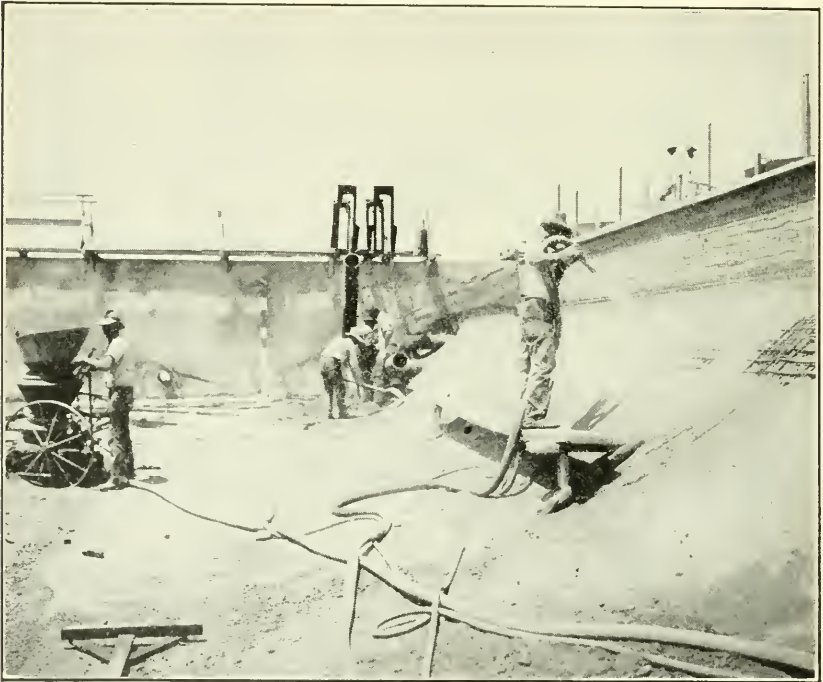
FIG. 23. Reinforced concrete construction of an oil sump, showing portion of one compartment.
