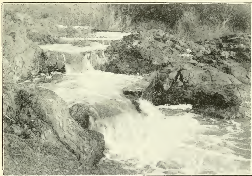
FIG. 20. Natural conditions utilized in the construction of a fishway. Note steelhead ascending in foreground.
