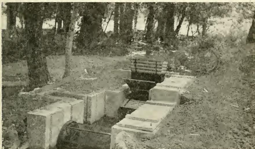
Looking upstream on a rotary fish screen. Power wheel in front of screen
