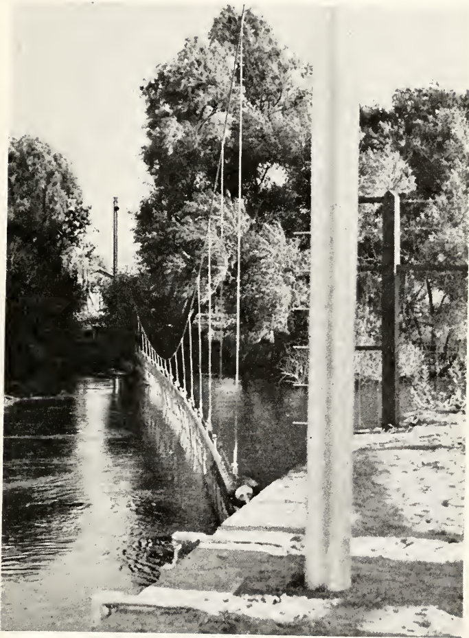
Figure 11. Experimental electric fish screen now being tested near Mendota. Photograph courtesy of Henry T. Burkly
