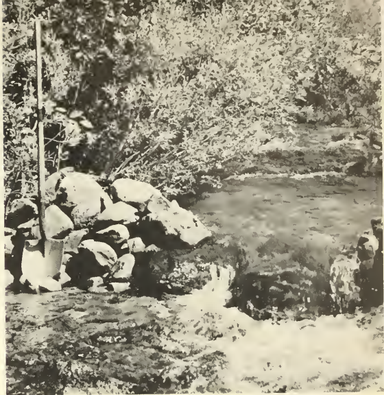
Typical rock deflectors constructed for flow maintenance and creation of natural pools for trout habitat.
