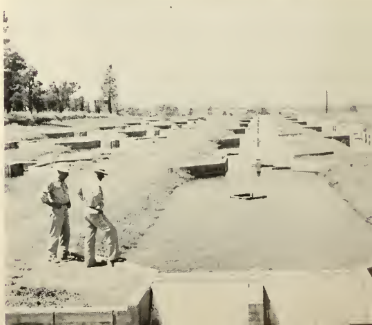
Rearing ponds at Darrah Springs Hatchery, largest trout installation in the State.
