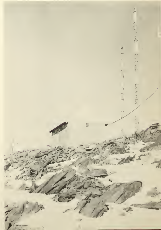
The radio repeater station at White Mountain, Inyo County, part of the communications network.
