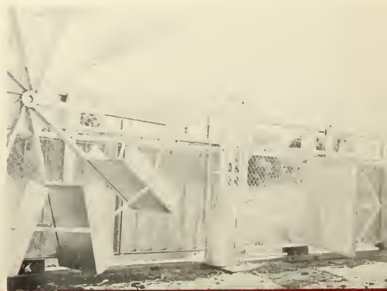
Newly designed fish screen for diversions, showing automatic gate in open position. The gate prevents loss of head in canal when debris has accumulated on screen.
