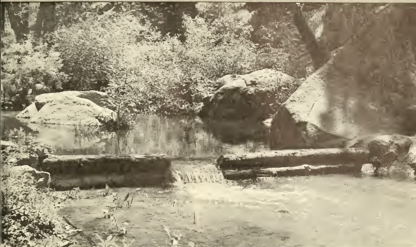
Lag dam built in 1954 by the department on Little Bear Creek, San Bernardino County, to create a trout pool. (Fish and Game Photo by B. H. Unruh)
