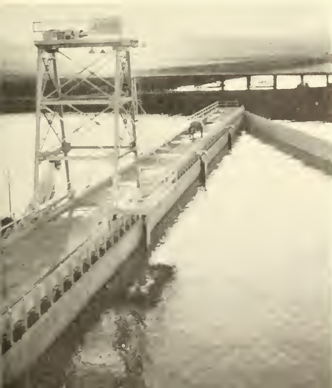
Fish screen at Tracy Pumping Plant of Delta Mendoto Canal on San Joaquin River.
